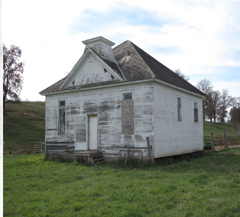
Photograph 1. Flowers School, looking southwest (October 2015)
